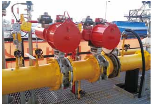
SK GAS - SK PDH PJT SHUT/OFF VALVE (TRIPLE OFFSET BFV-12")
